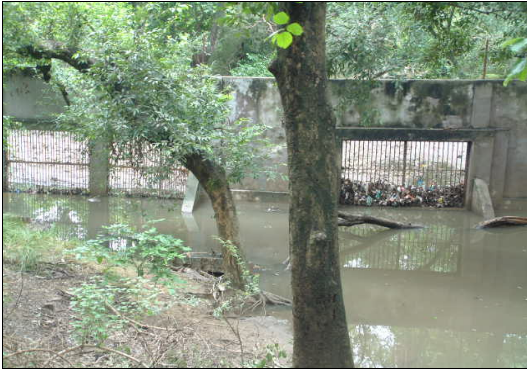
Figure 1 Water inlets--requires proper maintenance
